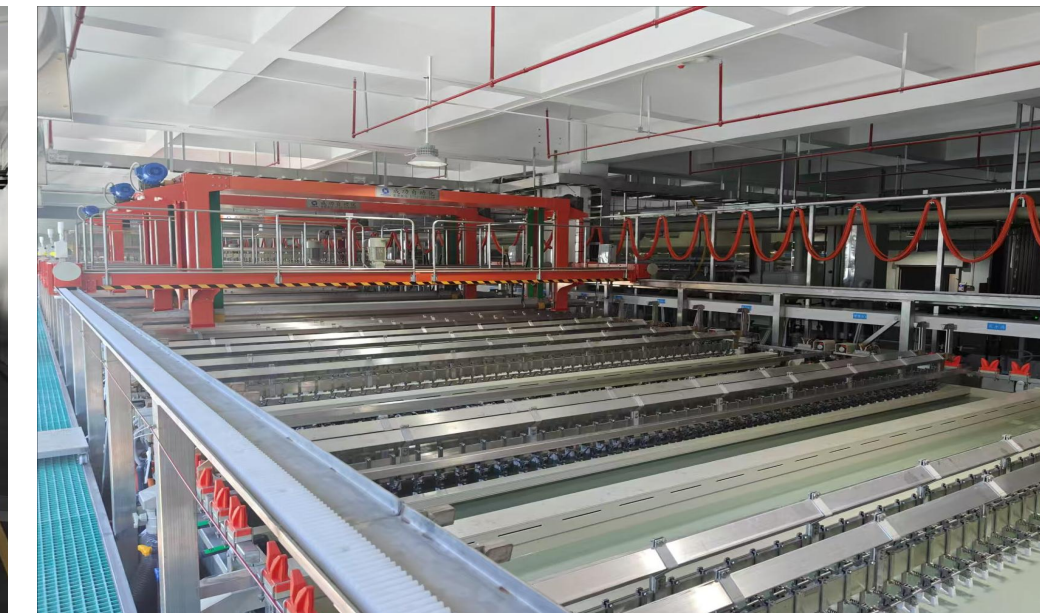
图形电镀线 Pattern Plating Line
